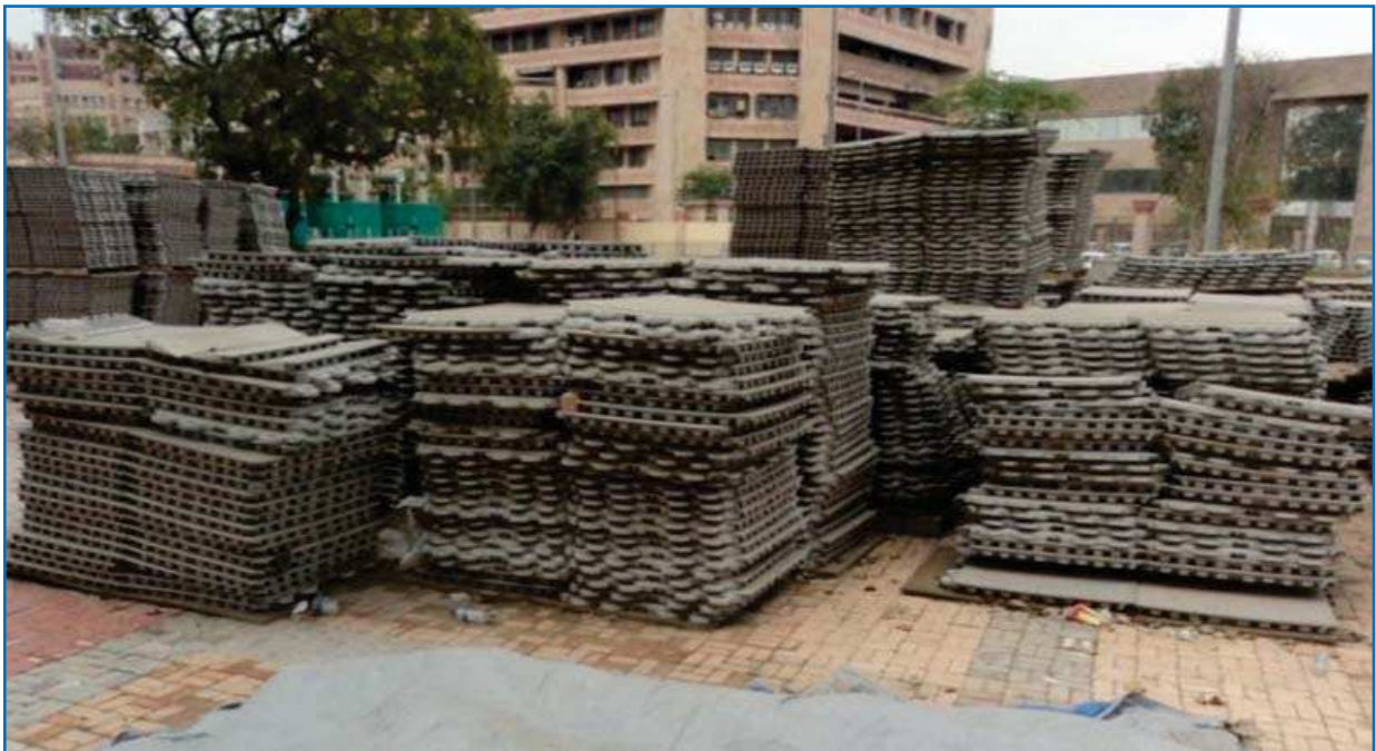
Unused Ground Protection Tiles (March 2011)
