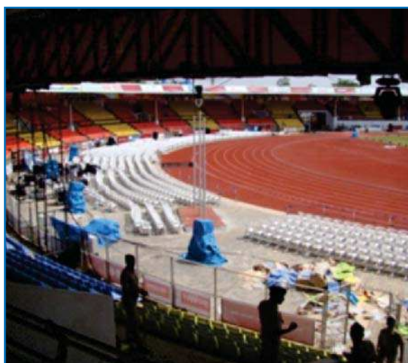
Renovated Athletic Stadium
