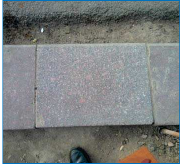
Granite kerb fixed at work site
