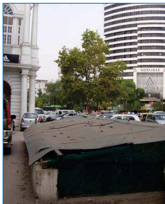
Covered subway entrance after re-filling
