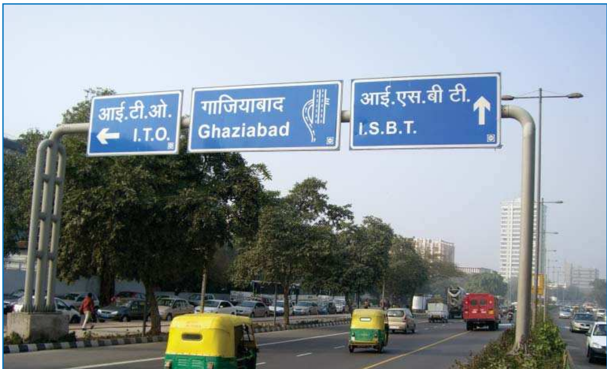
Cantilever mounted signage
