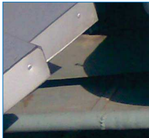
Riveting of ACM to frame
