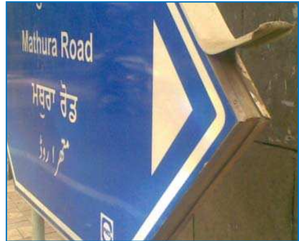
Aluminium Trim peeling off from frame
