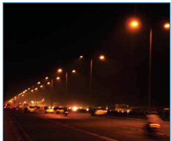
Modernised Street Lighting in Delhi
