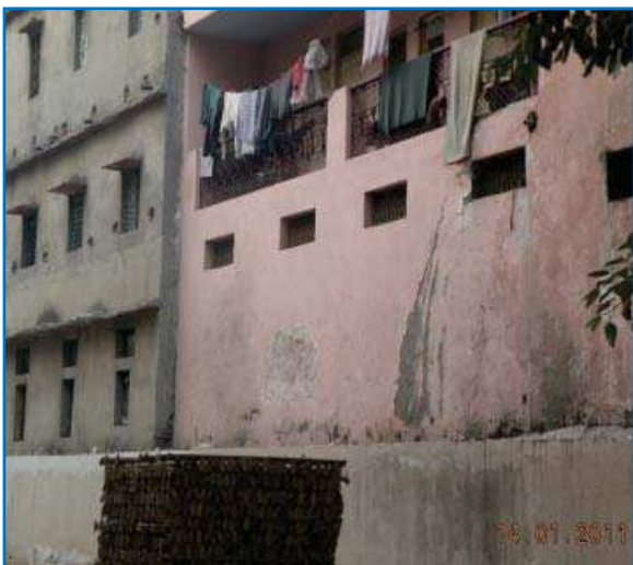
SRCC - Boundary Wall
