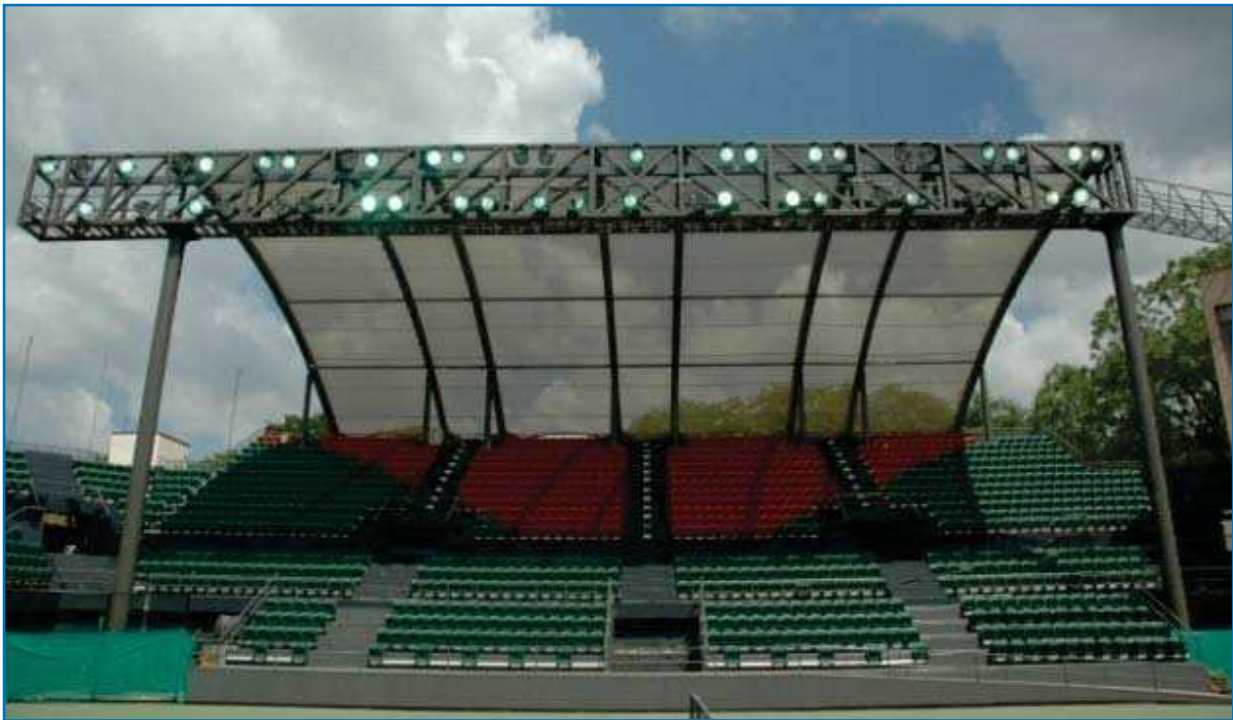
Centre court after renovation
